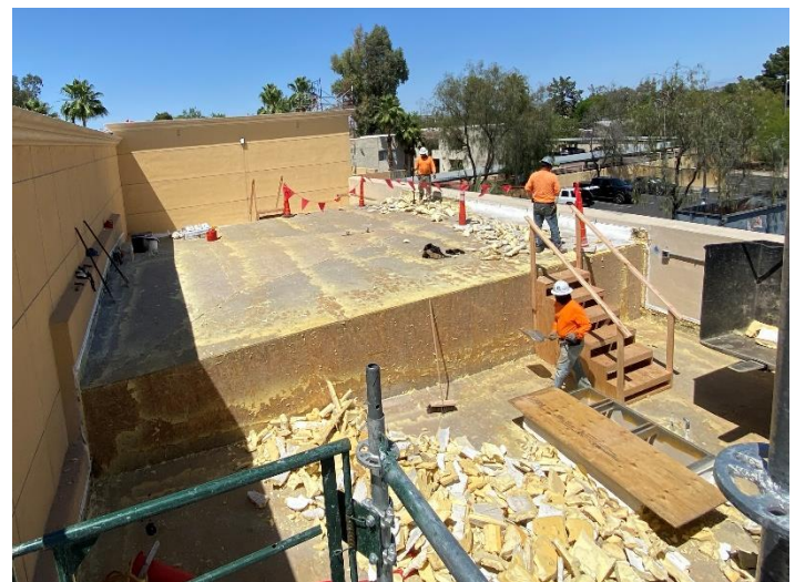
Roof Demo/Tear-off
