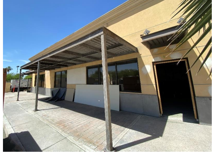
Prepped Steel Canopies for Paint
