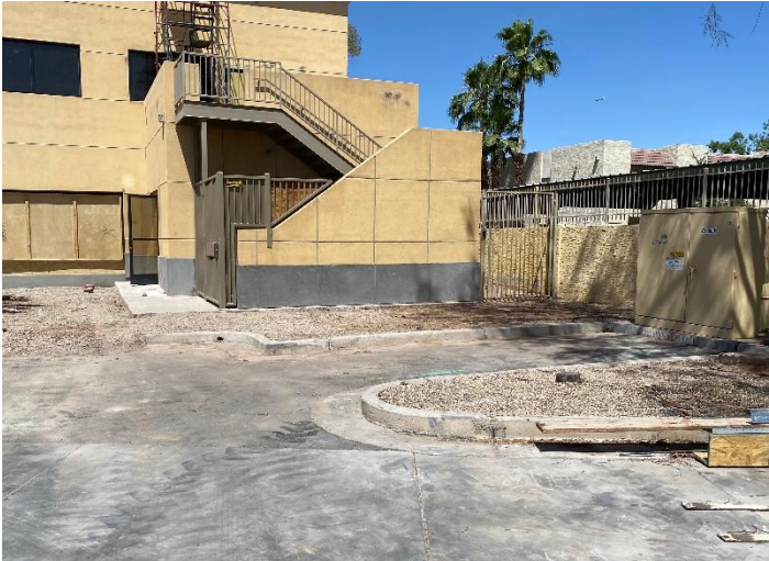
Grease Interceptor & Tallow Bin Removal
